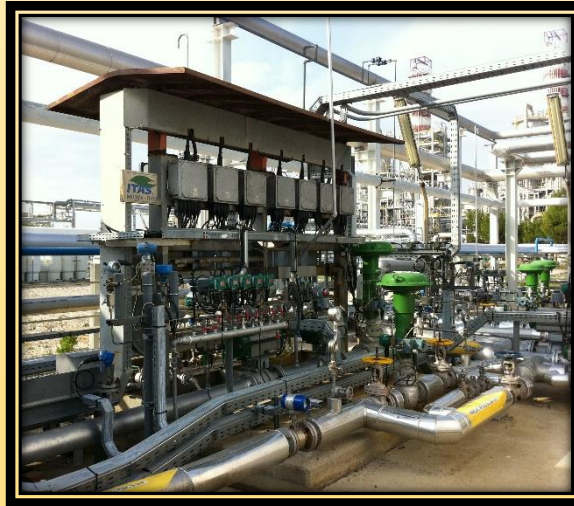
NEW CONTROL SYSTEM
