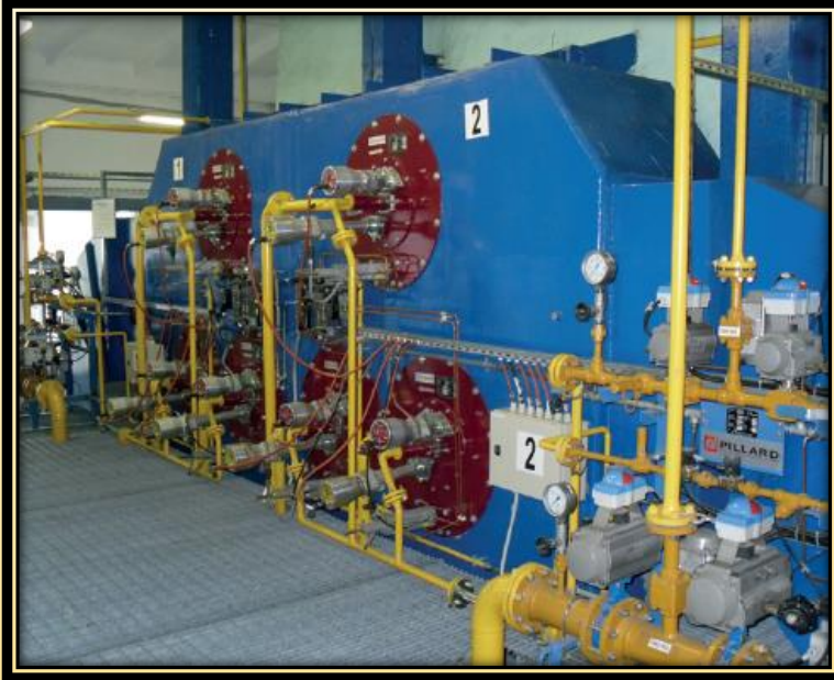
UTILITY BOILER BURNERS
